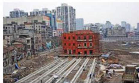
Fig.2: Relocation of a Building
